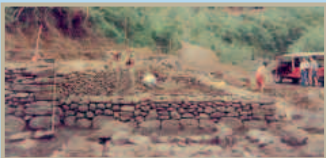
Travaux de restauration de Fare Hape - © SCP
